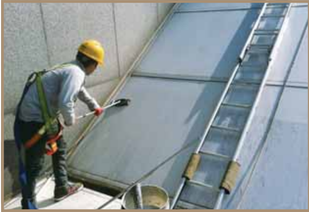
Training on Use of Fall Arrestor System
