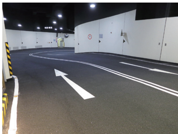
Carborundum Refurbishment at Car Park Driveway
