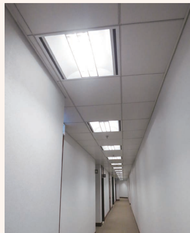
Retrofit of Fluorescent Luminaries to LED Lights
