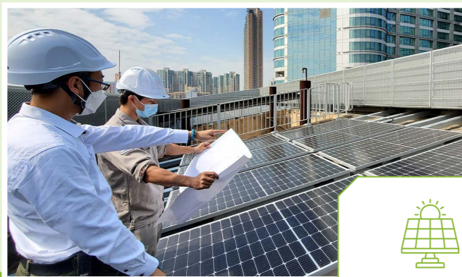
Rooftop solar panels
