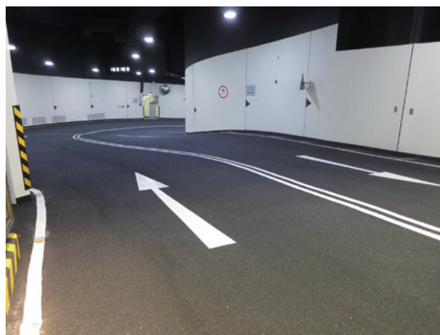
Carborundum Refurbishment at Car Park Driveway
